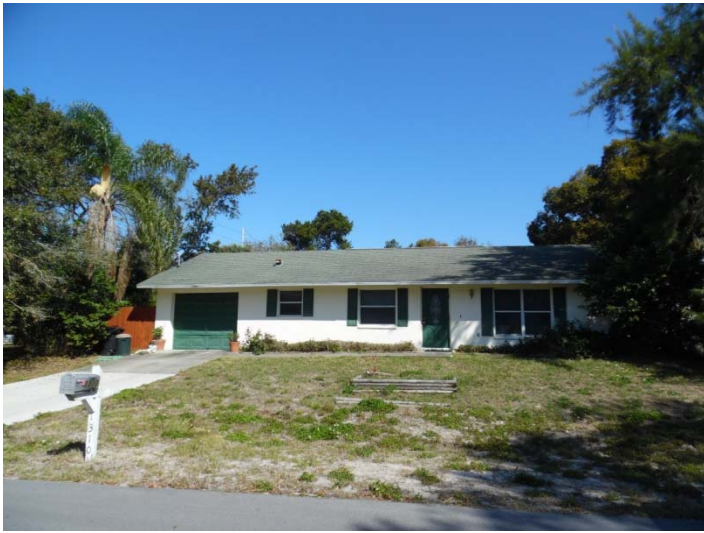
View looking north at the subject property, 1310 Idlewild Drive
