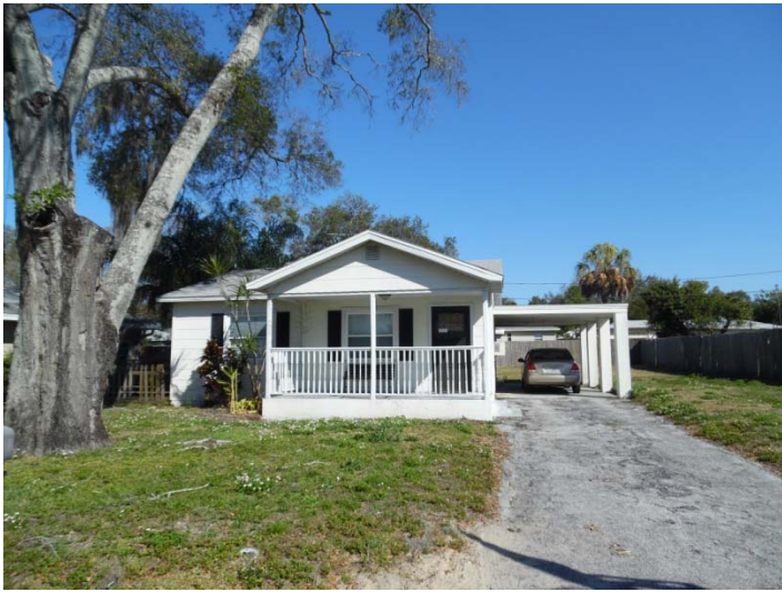
View looking north at the subject property, 1212 Sheridan Road
