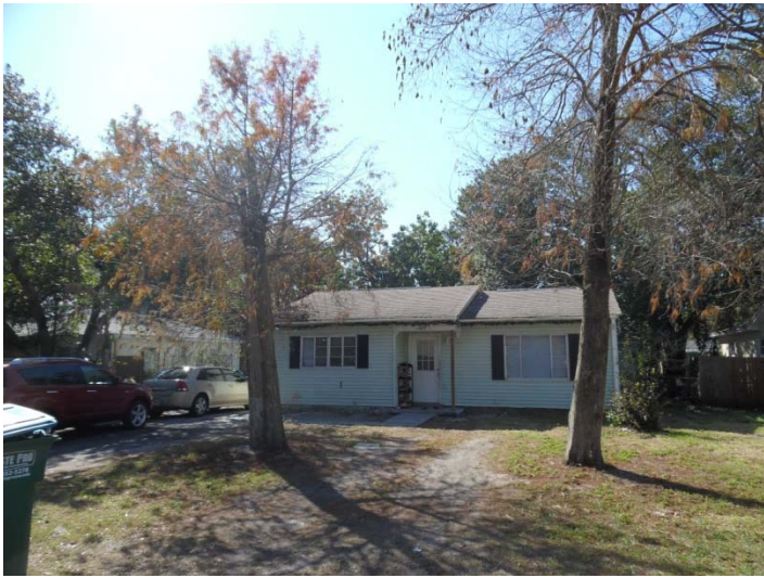
View looking south at the subject property, 1227 Union Street
