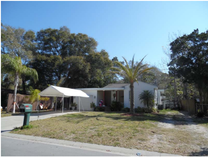
View looking east at the subject property, 2049 Poinsetta Avenue
