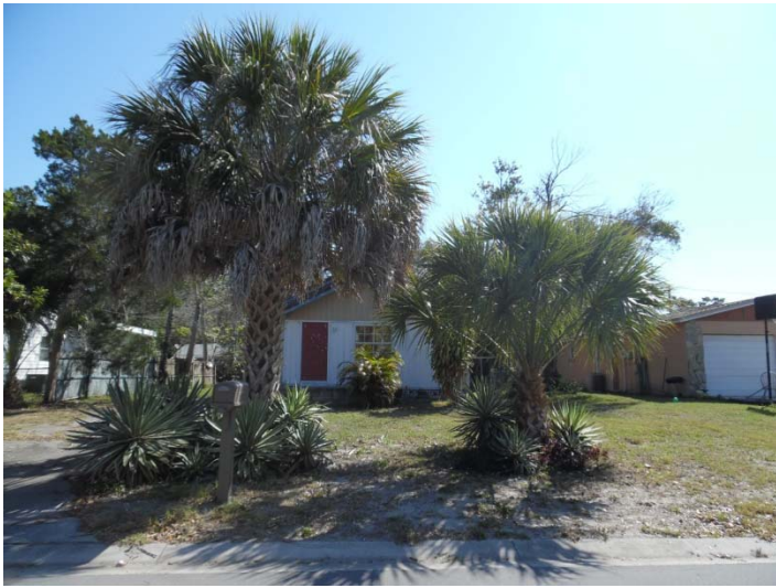
View looking east at the subject property, 2047 Poinsetta Avenue
