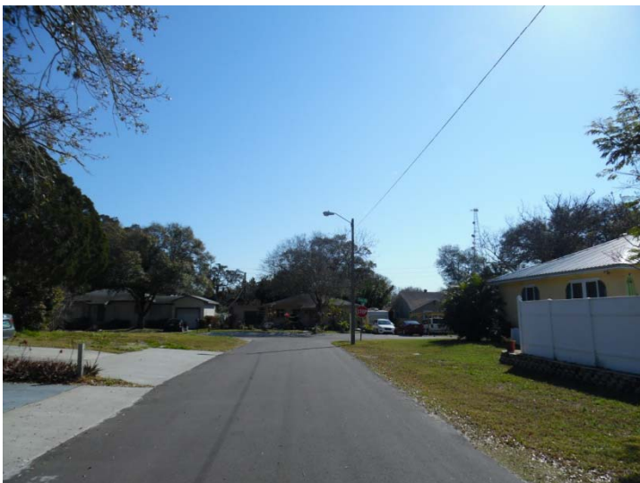
View looking easterly along Sheridan Road
