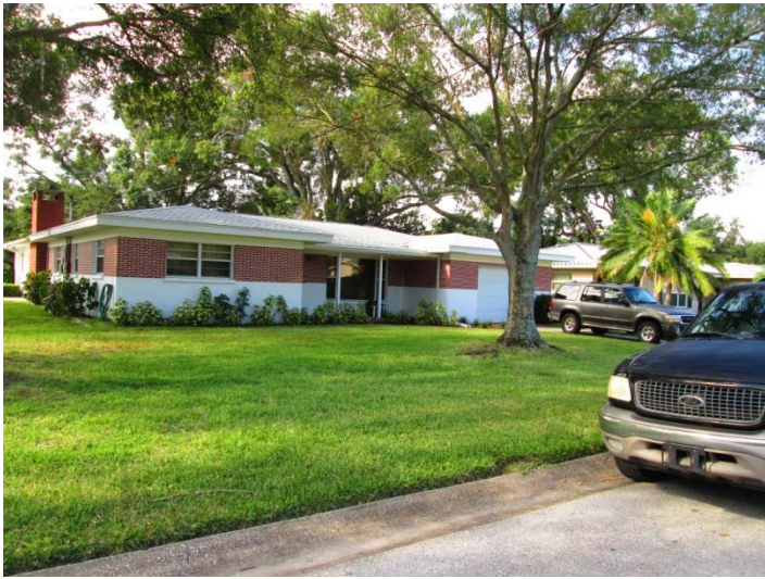
View looking south at the subject property, 3061 Glen Oak Avenue North
