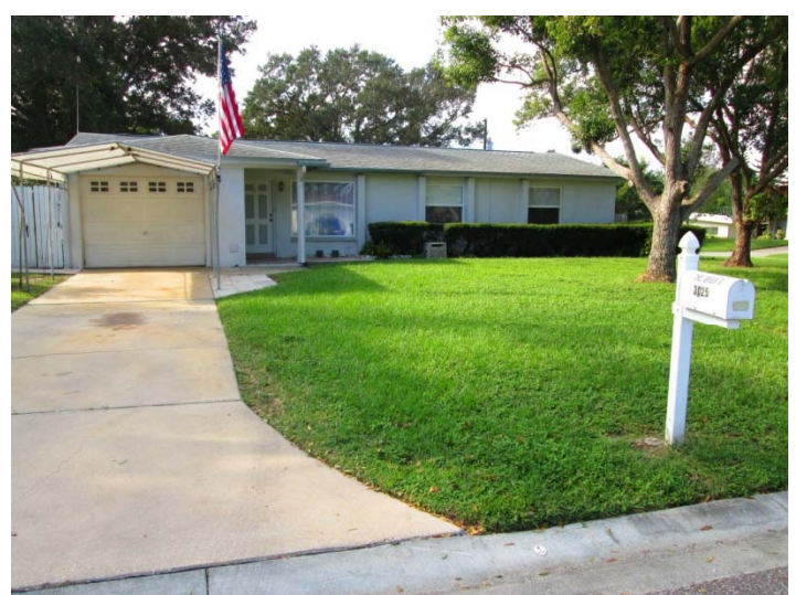
View looking south at the subject property, 3025 Glen Oak Avenue North
