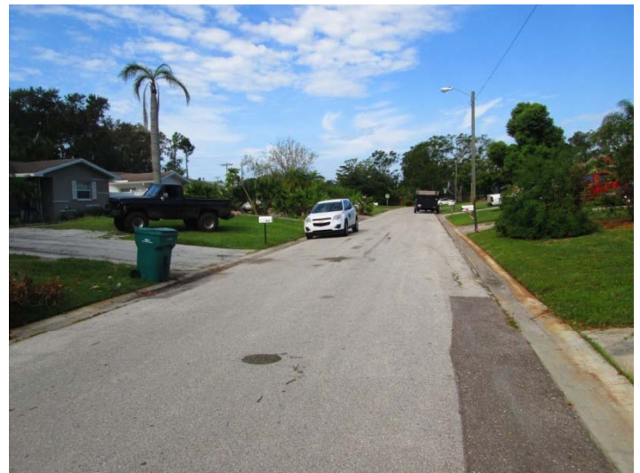
View looking westerly along Hoyt Avenue
