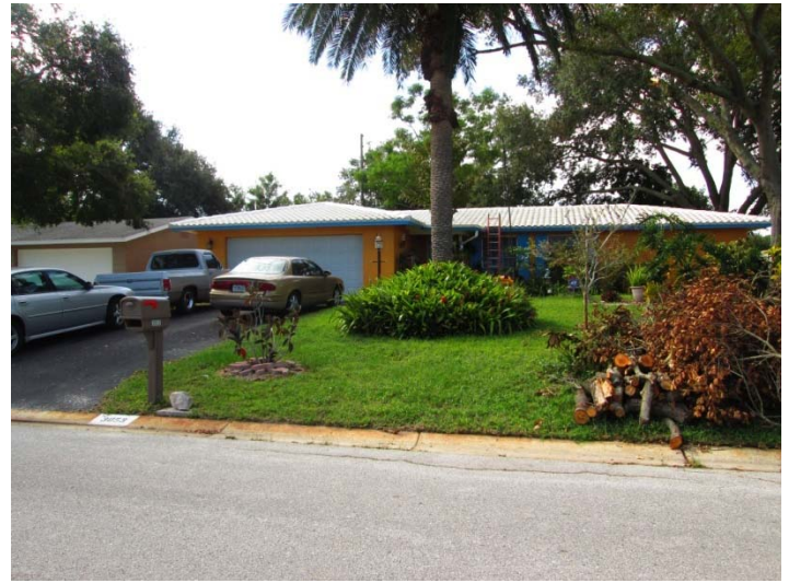
View looking south at the subject property 3053 Hoyt Avenue
