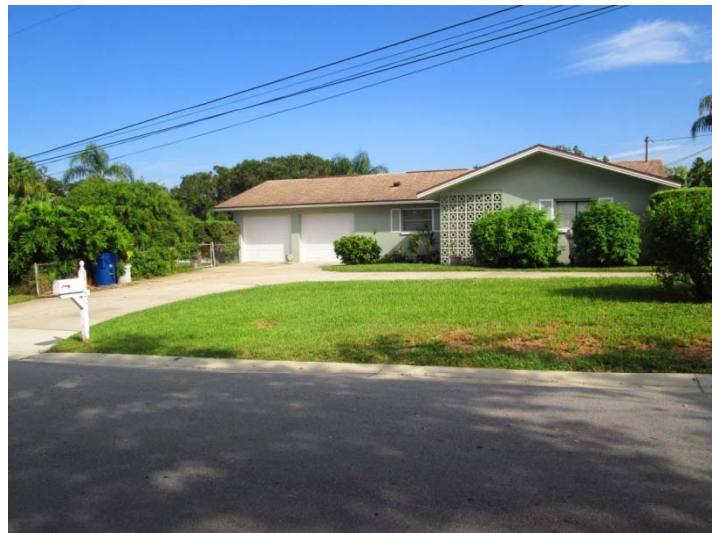
View looking north at the subject property, 3026 Grand View Avenue
