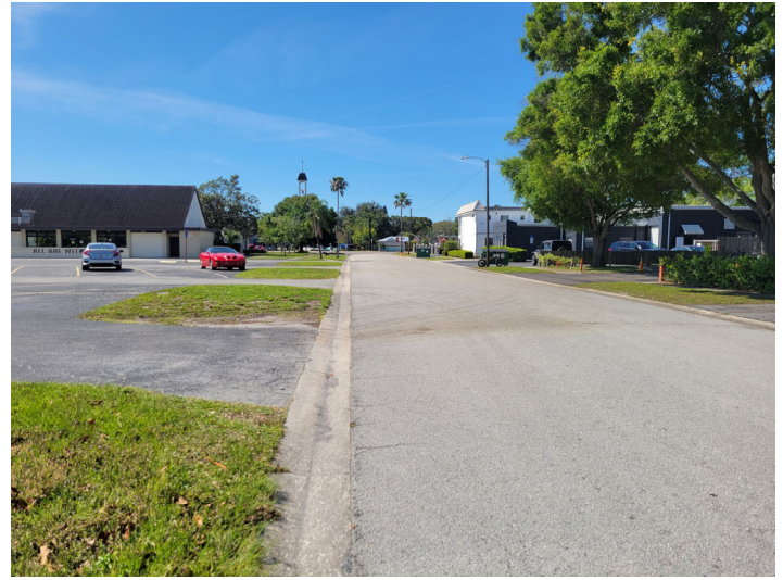
View looking southerly along S Saturn Avenue
