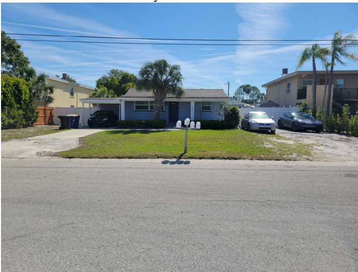
Across S Mars Avenue to the east
