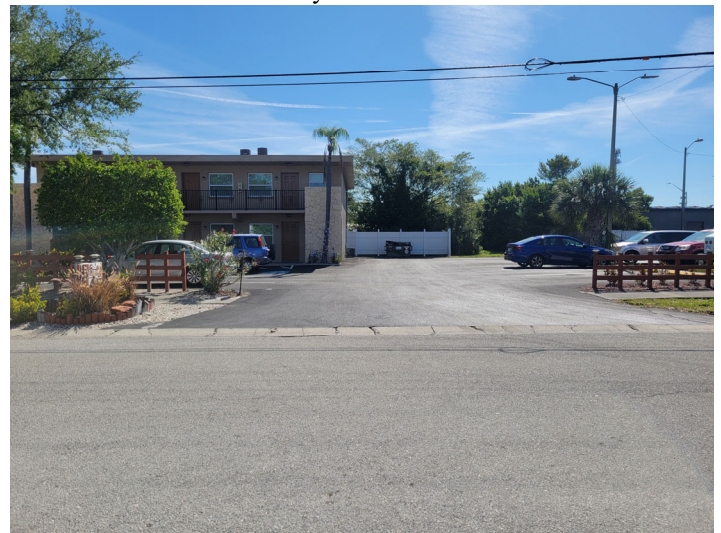
Across S Mars Avenue to the east
