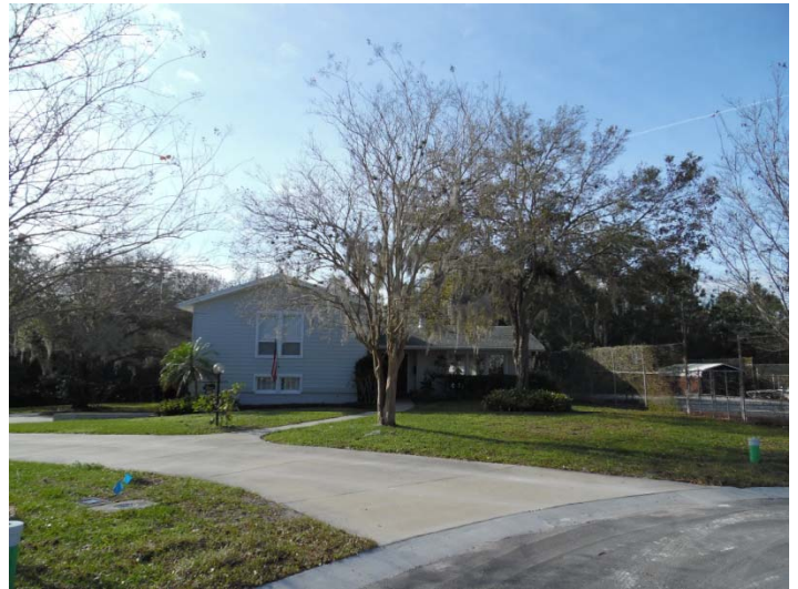
South of the subject property
