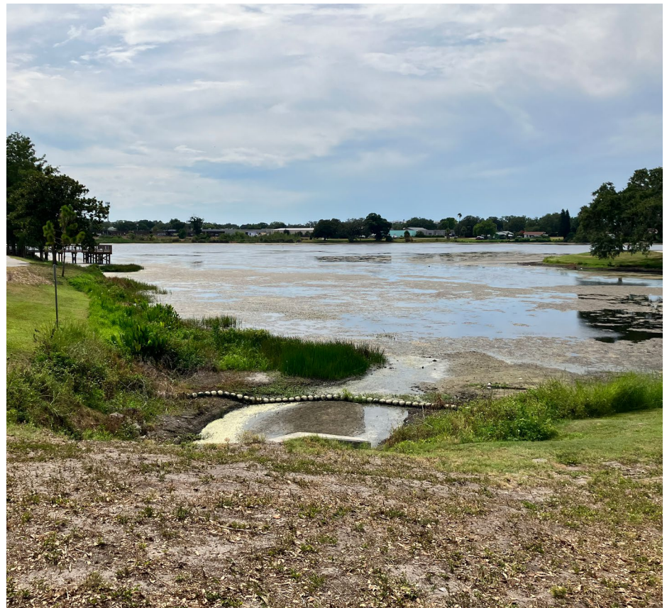
WATERGOAT stormwater system at Lake Belleview
