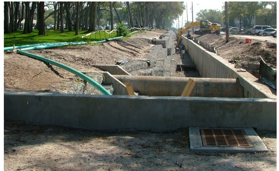
Construction of a stormwater system
