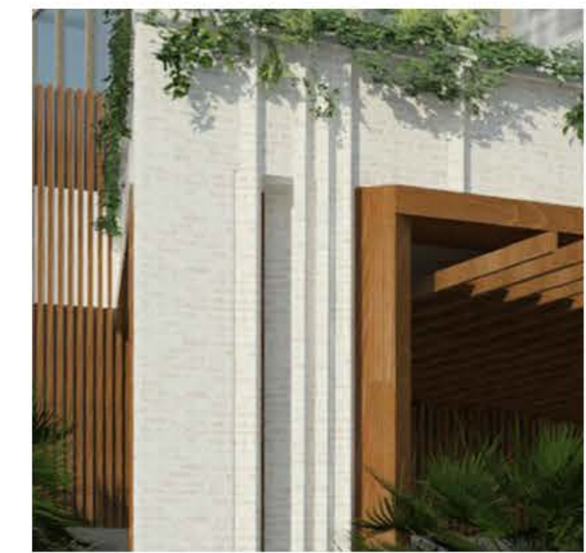
2) WHITE-WASHED BRICK CLADDING
