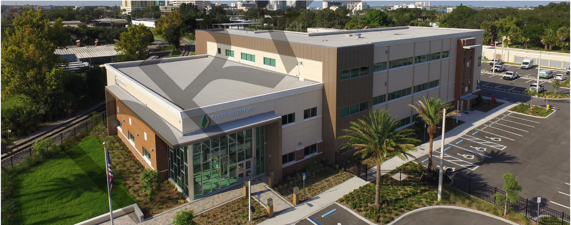
Clearwater Gas Administration Building
