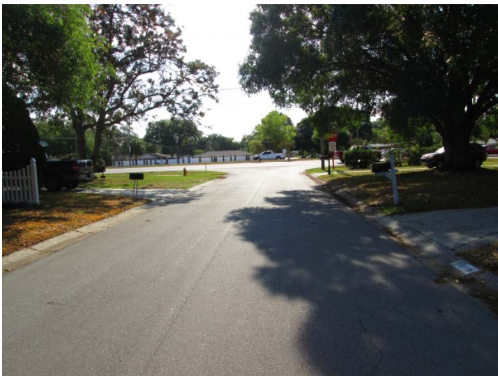
View looking easterly along Grand View Avenue
