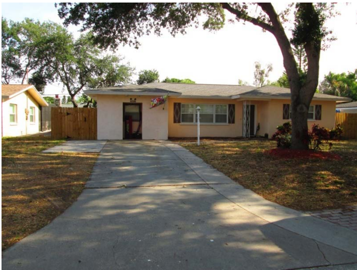
West of the subject property
