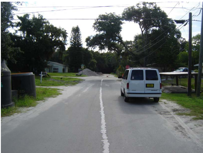
View looking easterly along Idlewild Drive
