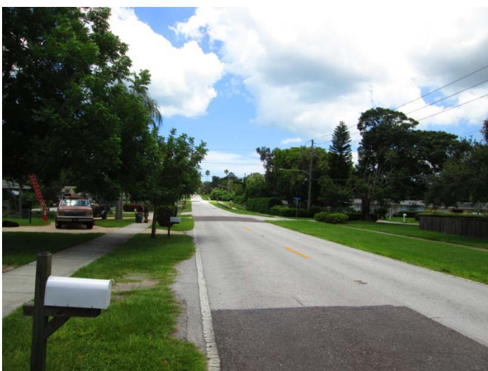
View looking westerly along Lakeview Road
