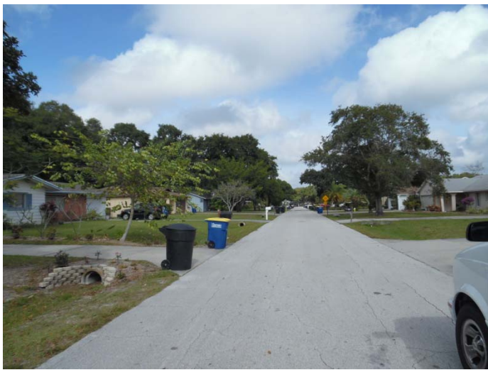
View looking northerly along Grove Drive
