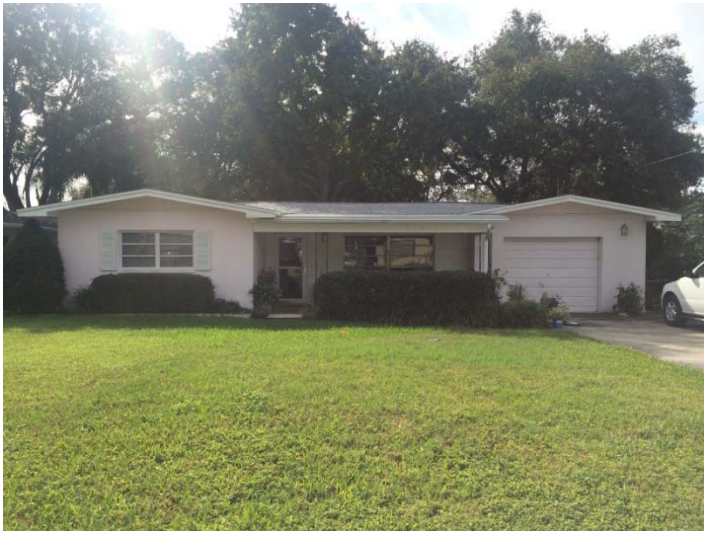
View looking south at the subject property, 2161 Burnice Drive
