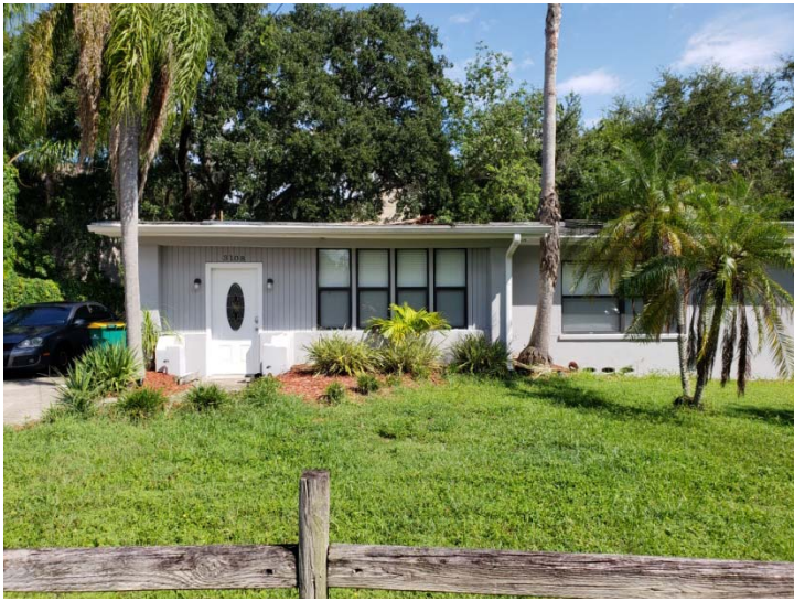
View looking north at the subject property 3108 Johns Parkway
