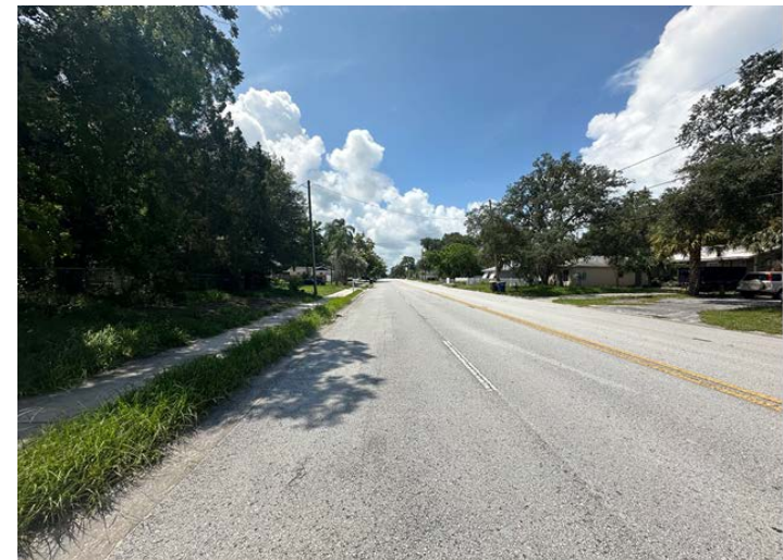
View looking southerly along Douglas Avenue
