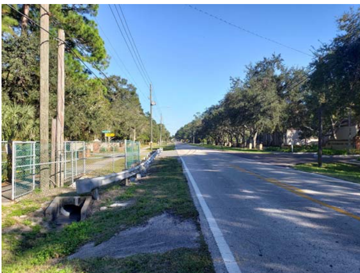
View looking easterly along Nursery Road
