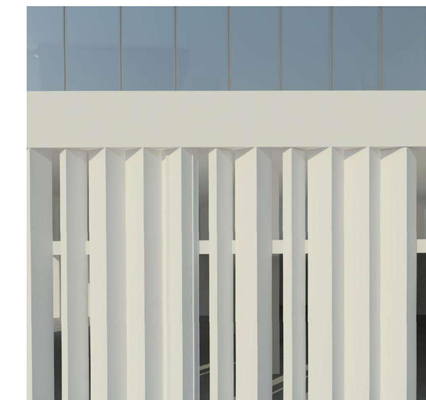
② VERTICAL CONCRETE PANELS
