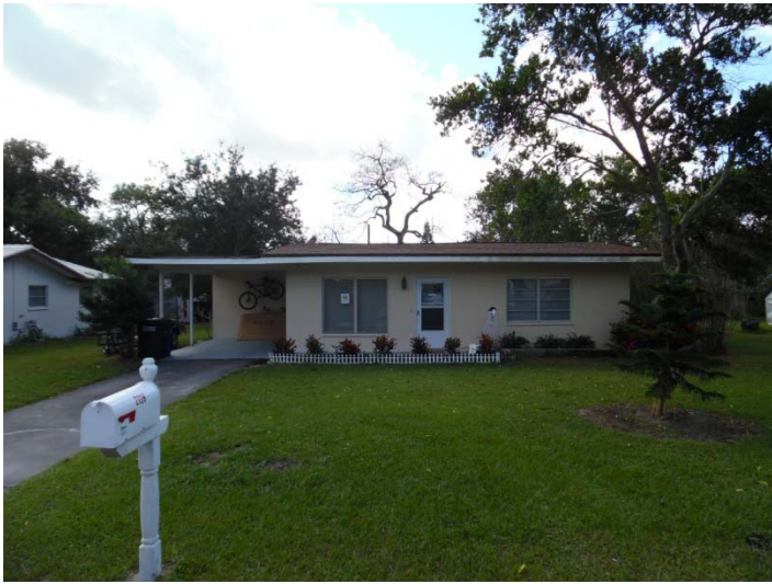
View looking south at the subject property, 2139 Bell Cheer Drive
