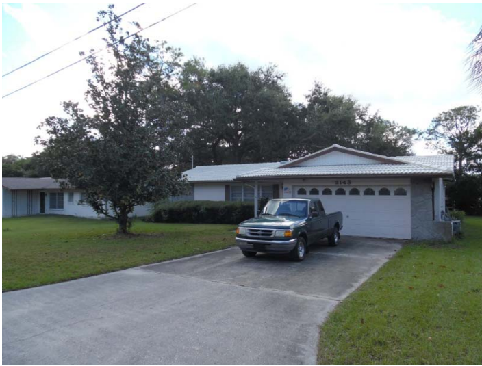
View looking south at the subject property, 2143 Bell Cheer Drive
