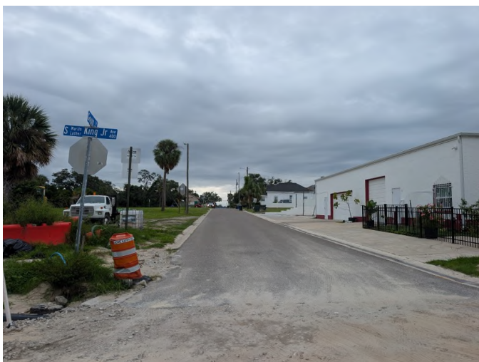
View Looking East Along Gould St
