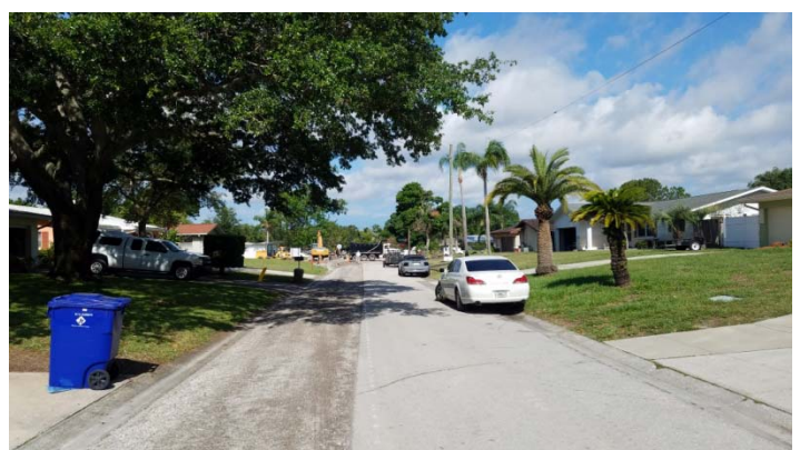
View looking westerly along Merrill Avenue
