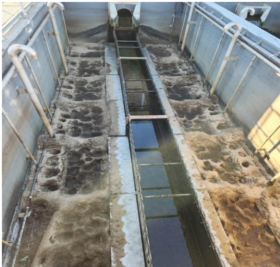
Cell #7 sand bed craters and voids
