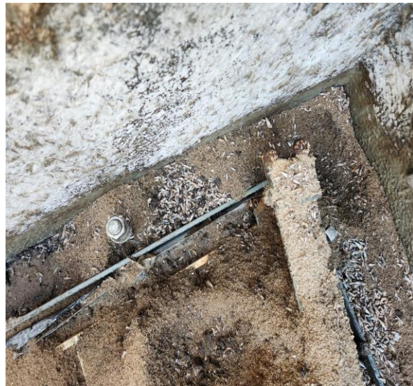
Cell #7 I-beam off holddown stud with tab missing
