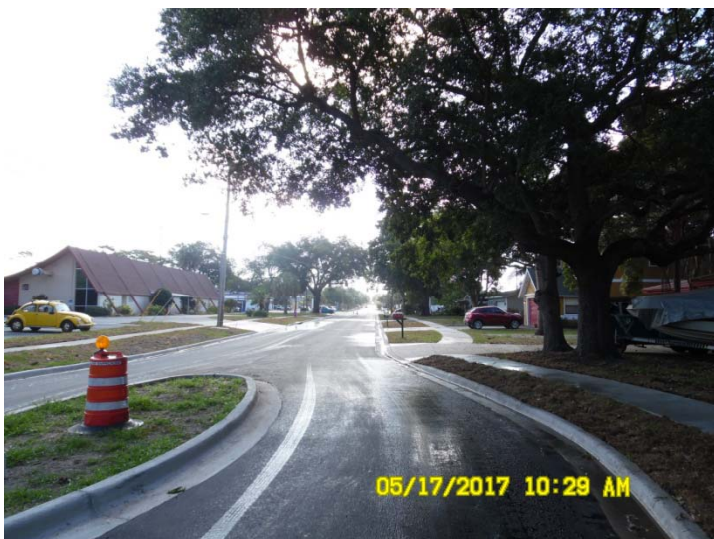
View looking easterly along Otten Street
