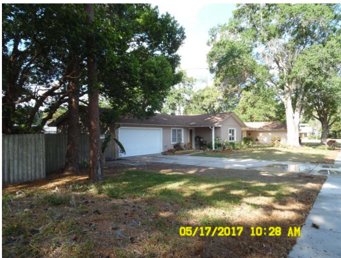
West of the subject property
