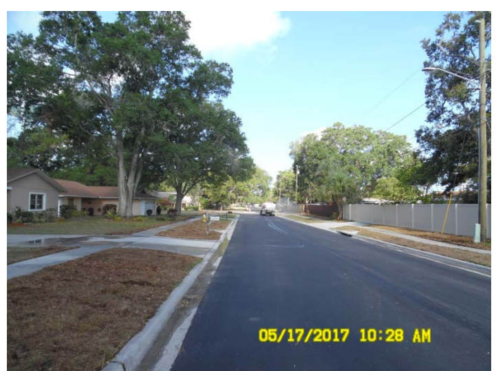
View looking westerly along Otten Street
