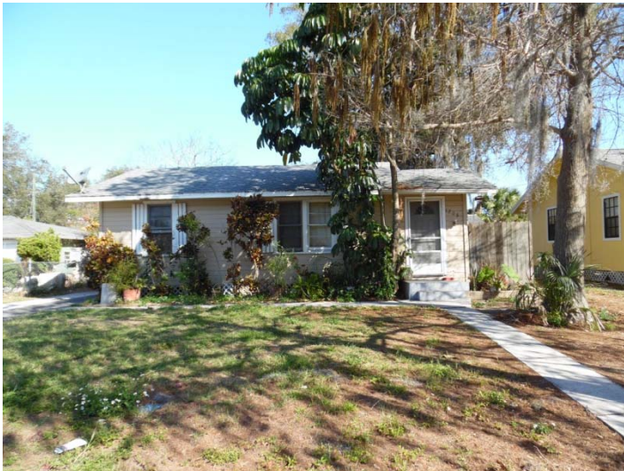
View looking north at the subject property, 1208 Sunset Point Road
