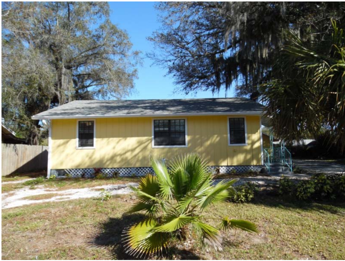
View looking north at the subject property, 1210 Sunset Point Road
