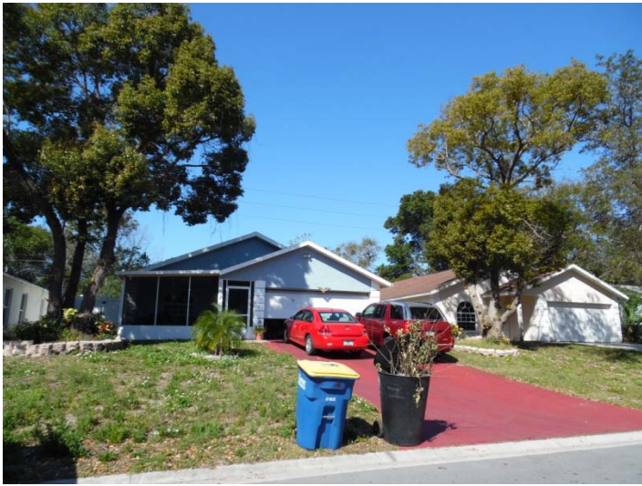
View looking west at the subject property, 2040 Poinsetta Avenue
