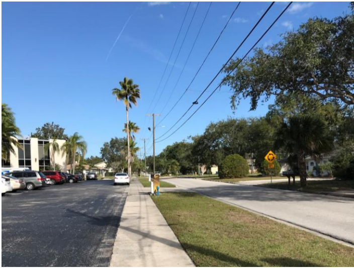
View looking northerly along South Duncan Avenue
