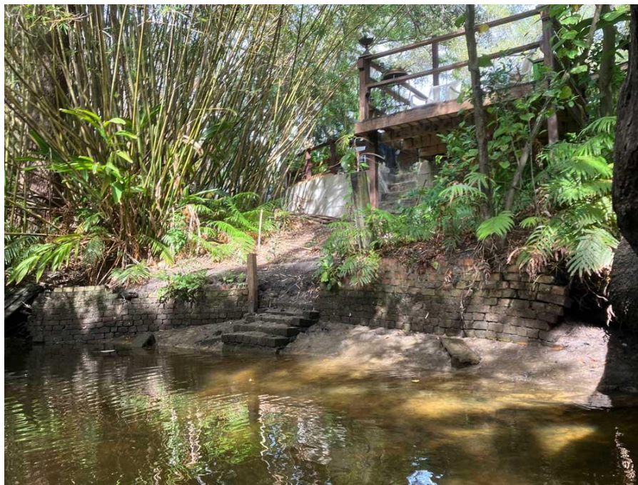
SUBJECT CREEKSIDE VIEW AT ELEVATED DECK
