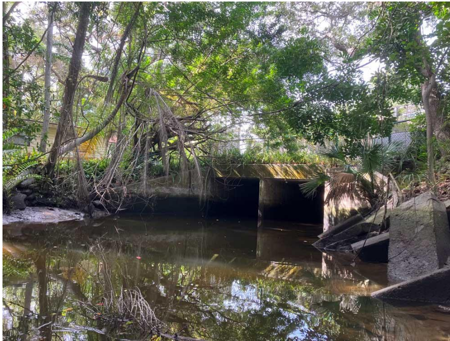
DOUGLAS AVENUE BRIDGE VIEW AT SUBJECT ON LEFT
