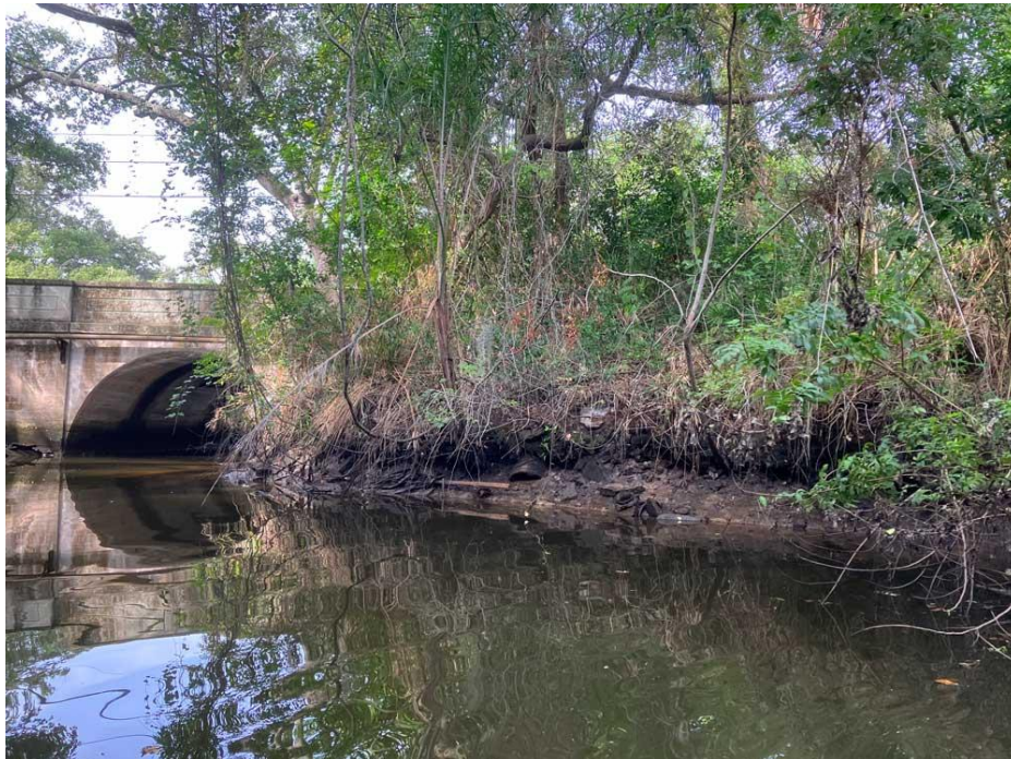
SPRINGTIME AVENUE BRIDGE VIEW AT SUBJECT ON RIGHT
