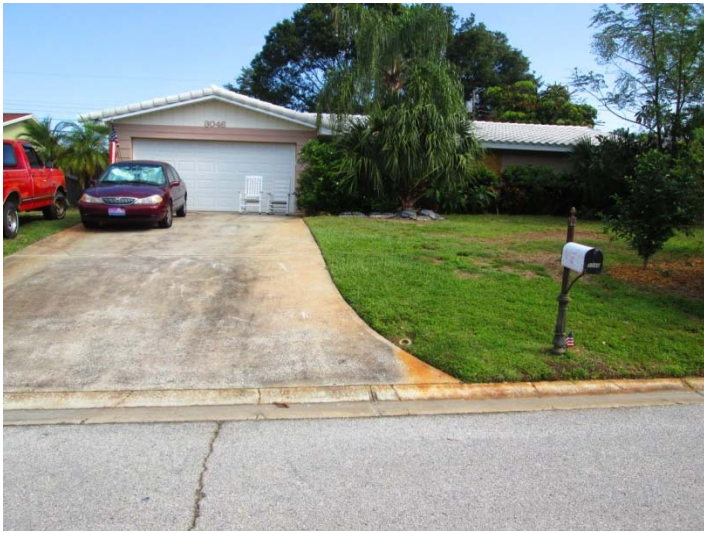
View looking north at the subject property 3046 Hoyt Avenue
