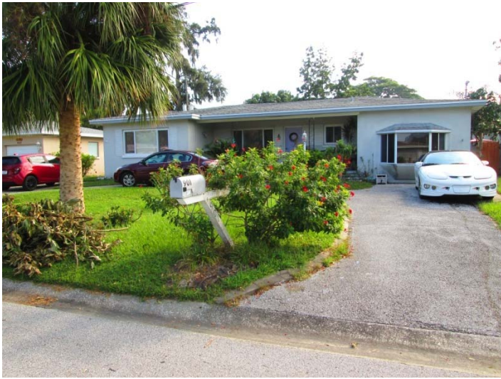
View looking east at the subject property, 901 Glen Oak Avenue East
