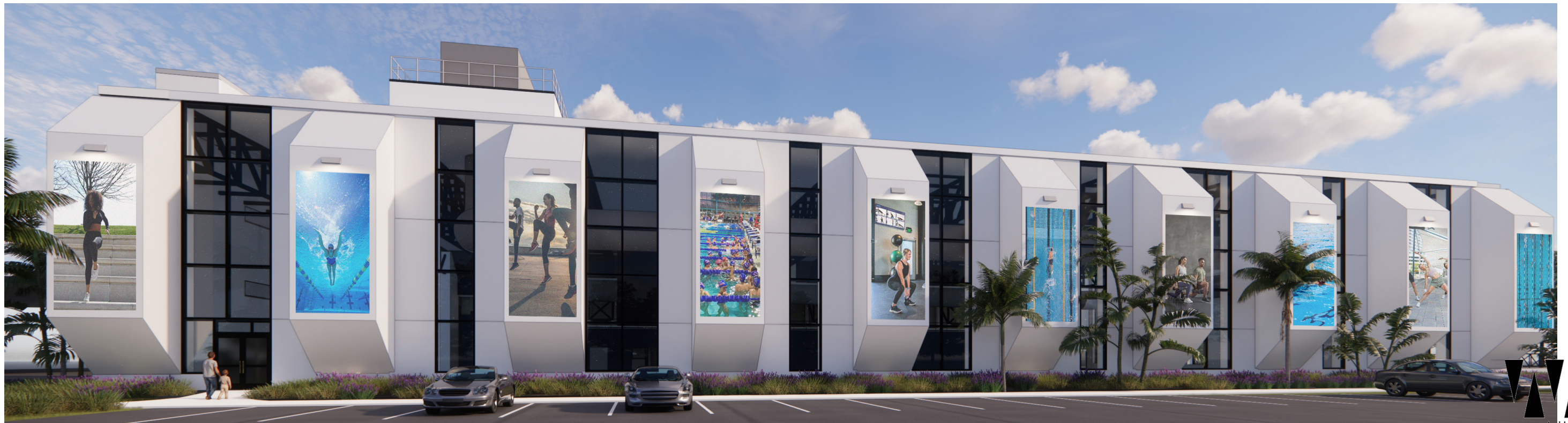
Exterior | North Facade
