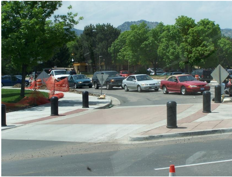
Figure 77 | Raised Crosswalk at Channelized Right Turn
