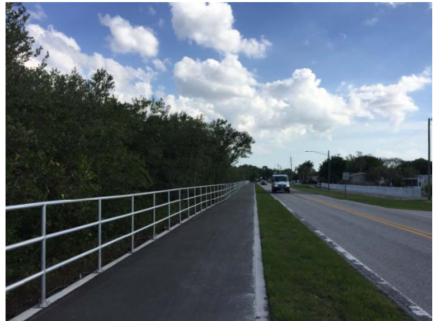
12. View looking southerly along Bayshore Drive at Johns Parkway
