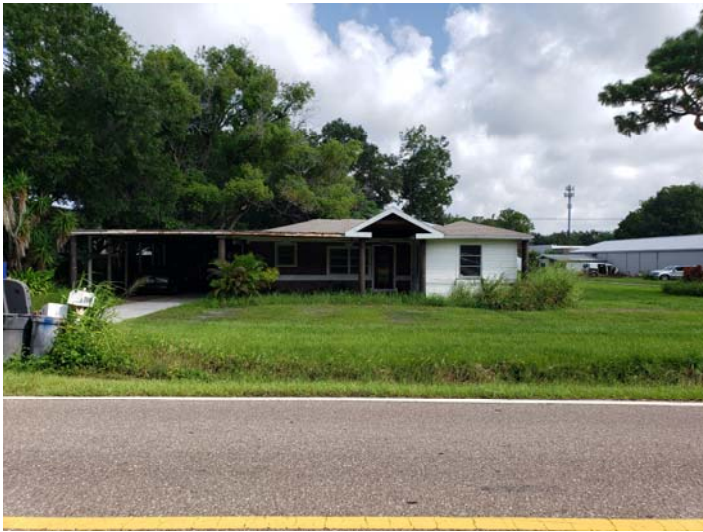
View looking north at subject property, 2108 Palmetto Street.
