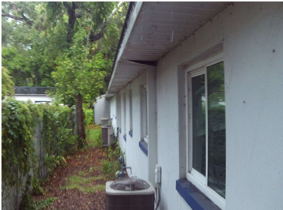
BUILDING 100, SOUTHERN ELEVATION, FACING WEST
