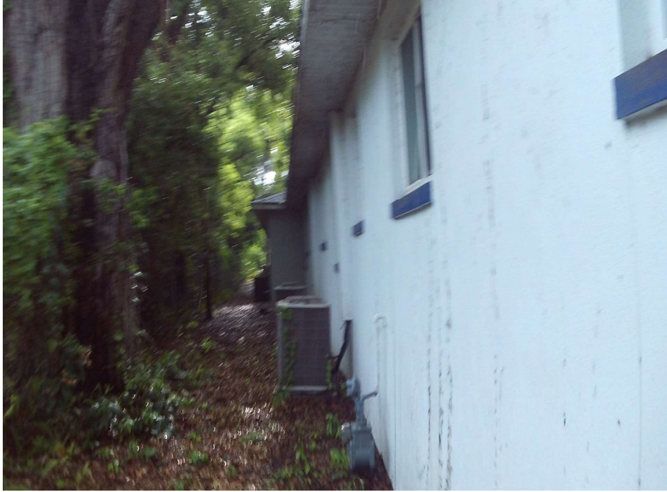
BUILDING 200, NORTHERN ELEVATION FACING EAST
