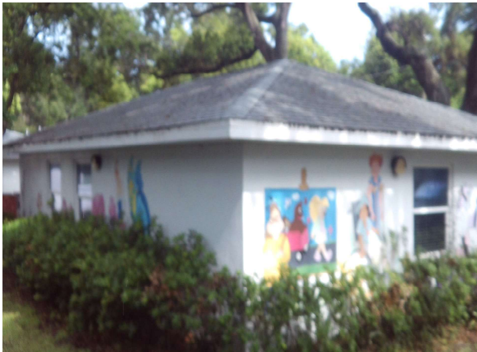
REAR VIEW, COMMUNITY CENTER
