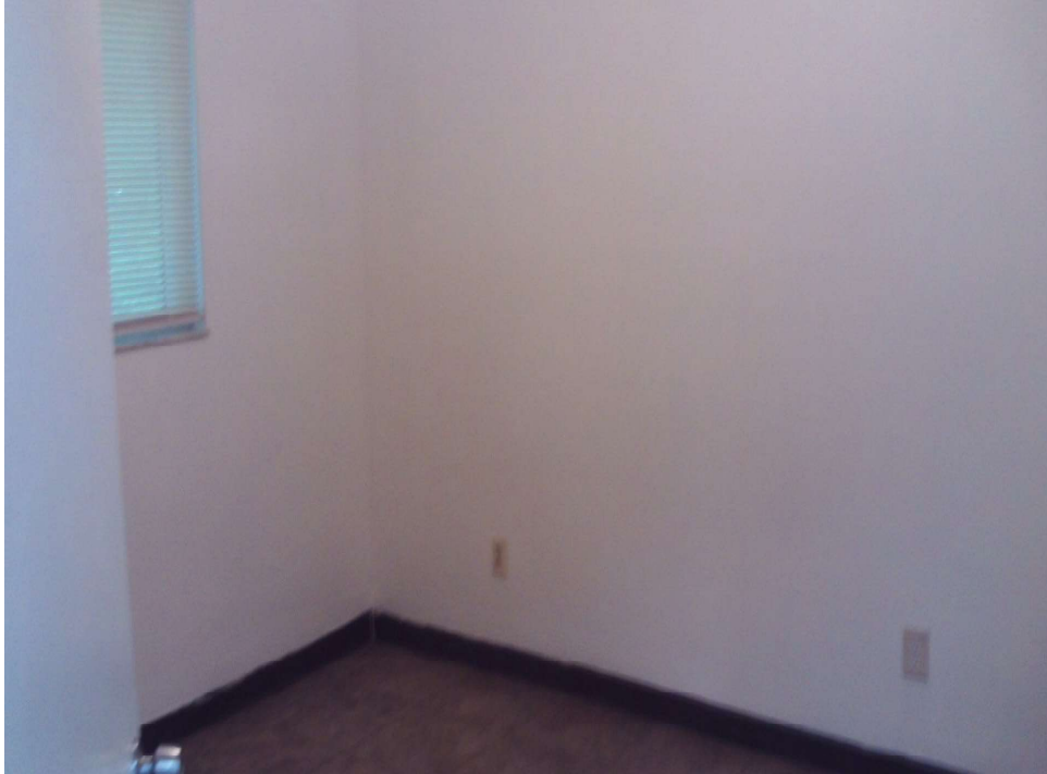
INTERIOR, UNIT 206 BEDROOM
