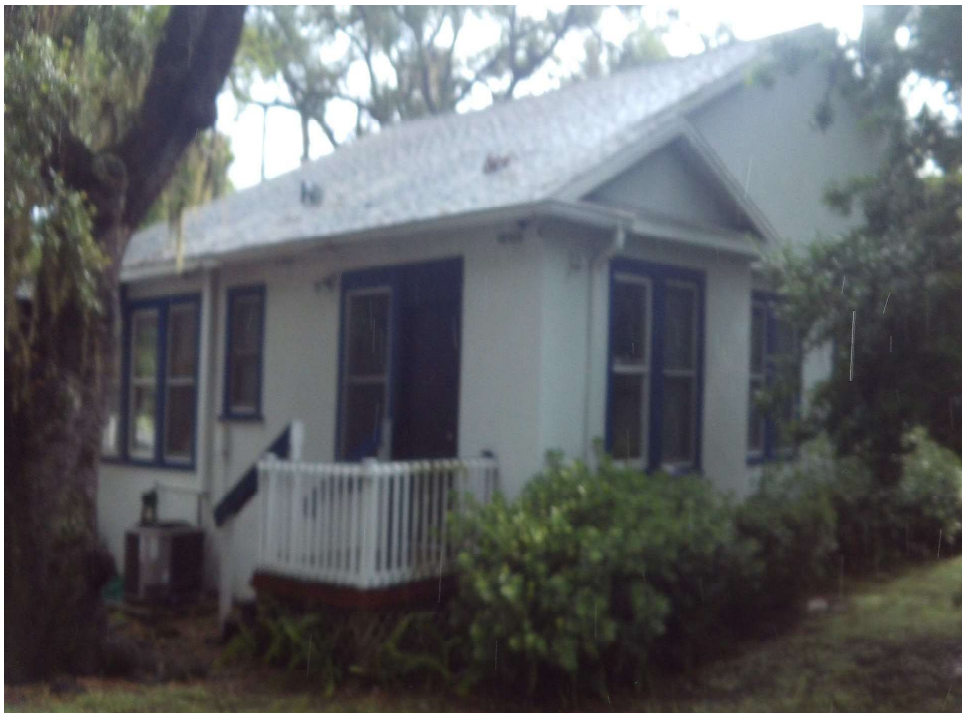
REAR AND SOUTHERN ELEVATIONS, OFFICE
