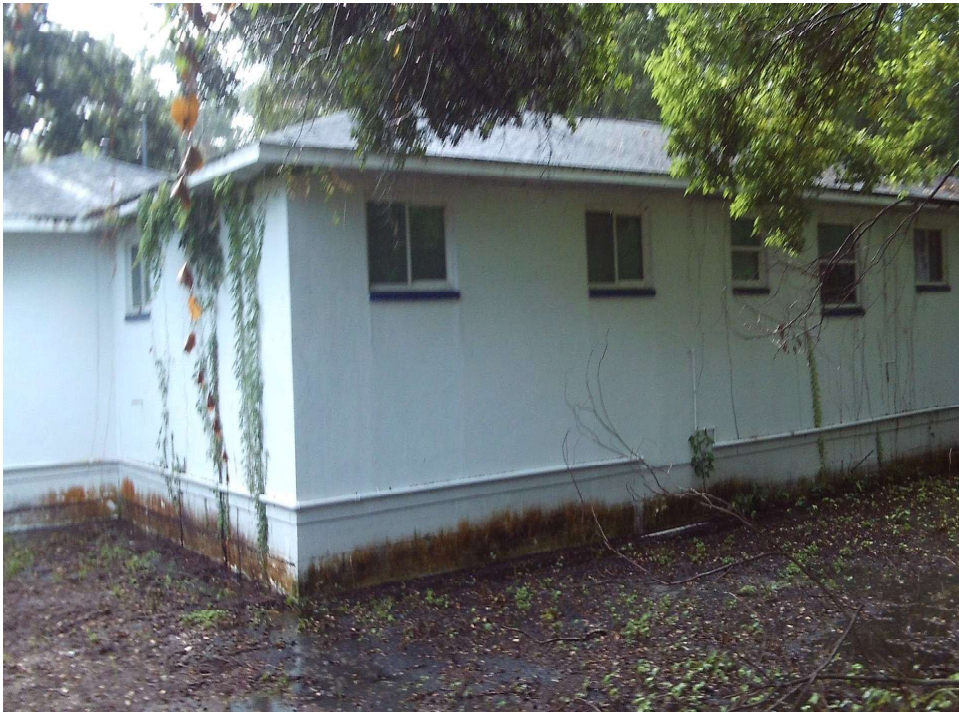
BUIDING 200, WESTERN ELEVATION, FACING SOUTHEAST
