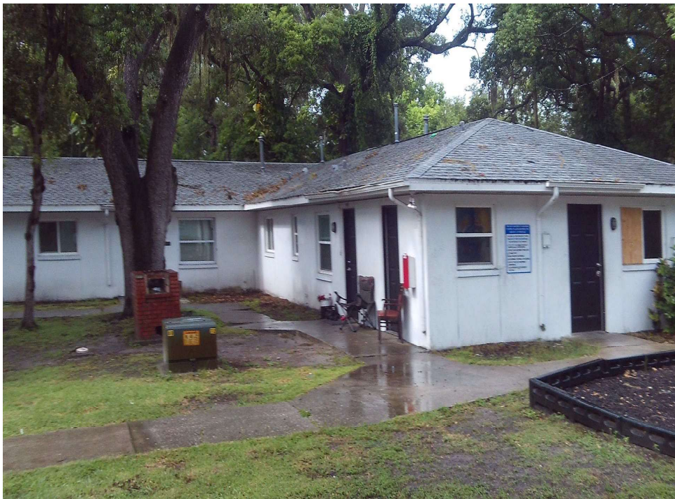
BUILDING 100, NORTHERN ELEVATION FACING SOUTH
