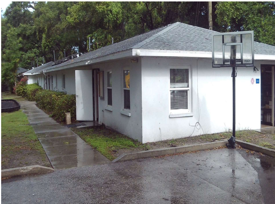
BUILDING 200, EASTERN AND SOUTHERN ELEVATIONS
