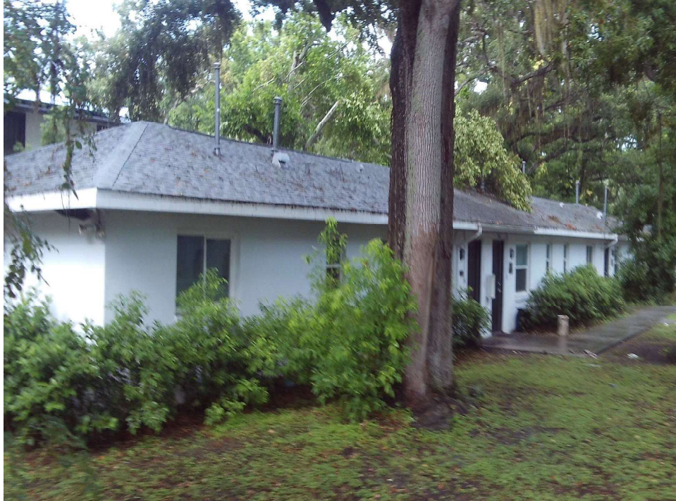
BUILDING 100, NORTHERN ELEVATION, FACING SOUTHWEST
