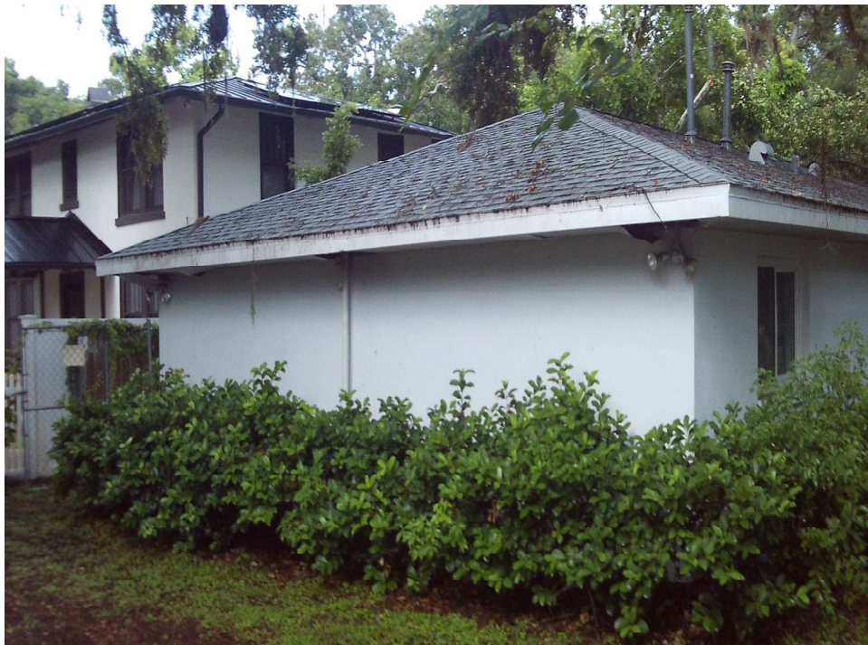
BUILDING 100, EASTERN ELEVATION, FACING SOUTHWEST
