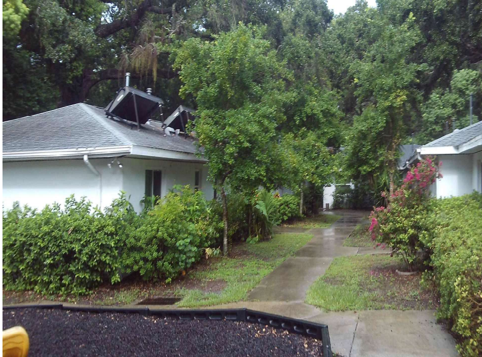
BUILDING 200, COURTYARD ACCESSING FRONTS OF UNITS, FACING WEST
