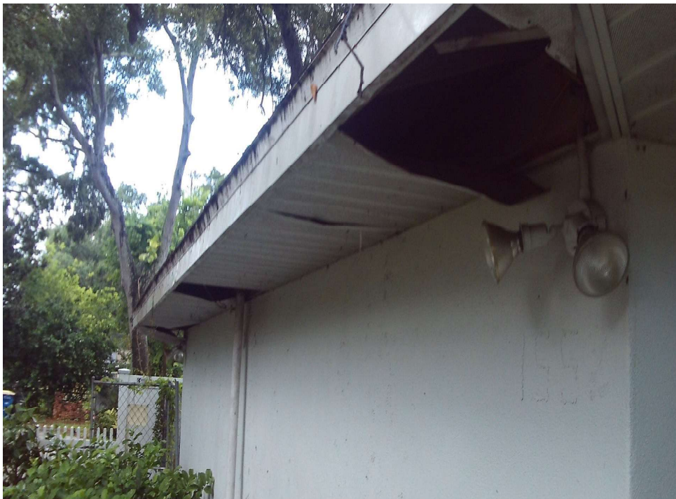
ALUMINUM SOFFITS, EASTERN ELEVATION OF BUILDING 100
