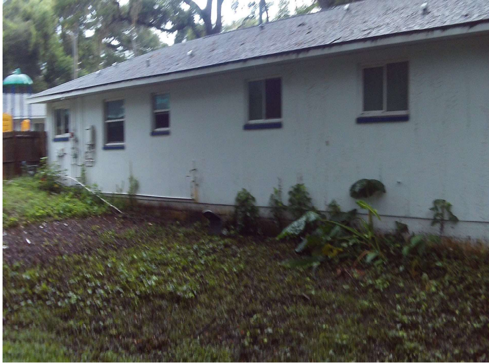
BUILDING 100, WESTERN ELEVATION, FACING NORTHEAST
