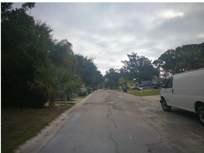
View looking easterly along Grand View Avenue
