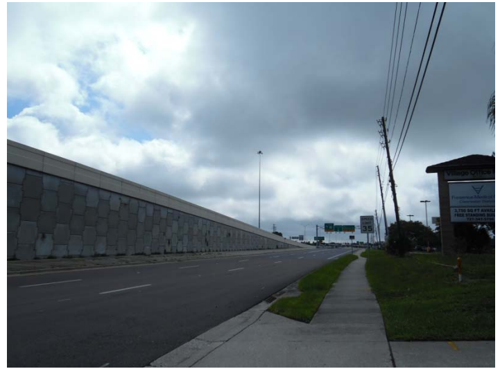
View looking southerly along US Highway 19 N
