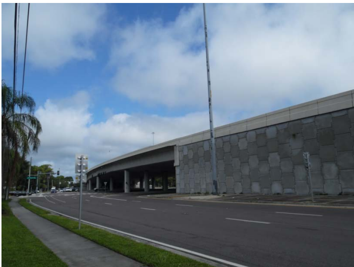
View looking northerly along US Highway 19 N Frontage Road
